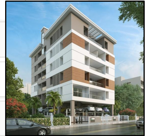
PROJECT : VIDURKRUPA DEVELOPER : GANGOTREE LOCATION : IDEAL COL. PROJECT AREA : 20,000SQFT STATUS : ONGOING
