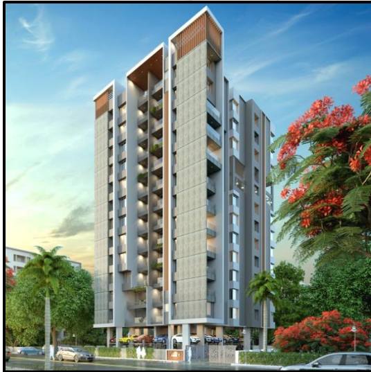
PROJECT : AYODHYANAGARI DEVELOPER : GOKHALE CO. LOCATION : DAHANUKAR COLONY PROJECT AREA : 56,000 SQFT STATUS : ONGOING
