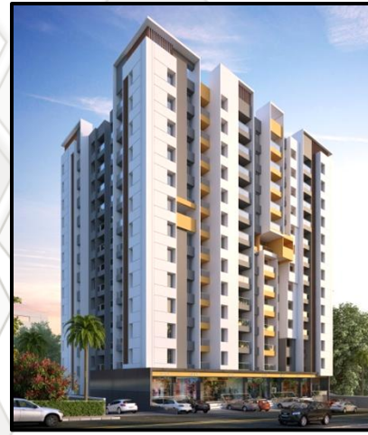
PROJECT : PUSHKAR PARK DEVELOPER : BHANDARI & ASSO. LOCATION : KOTHRUD PROJECT AREA : 95,000 SQFT STATUS : ONGOING
