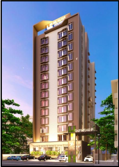
PROJECT : SNEHSHILP DEVELOPER : BELVALKAR HSG. LOCATION : DAHANUKAR COL. PROJECT AREA : 23,500SQFT STATUS : ONGOING
