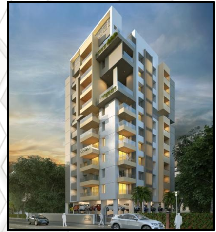
PROJECT : ANUPRITA 'B' DEVELOPER : GOKHALE CO. LOCATION : DAHANUKAR COLONY PROJECT AREA : SQFT STATUS : ONGOING
