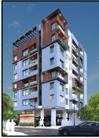
PROJECT : MAHESH SOCIETY DEVELOPER : OMKAR DHANKAWDE LOCATION : BIBWEWADI PROJECT AREA : 20,300 SQFT STATUS : ONGOING
