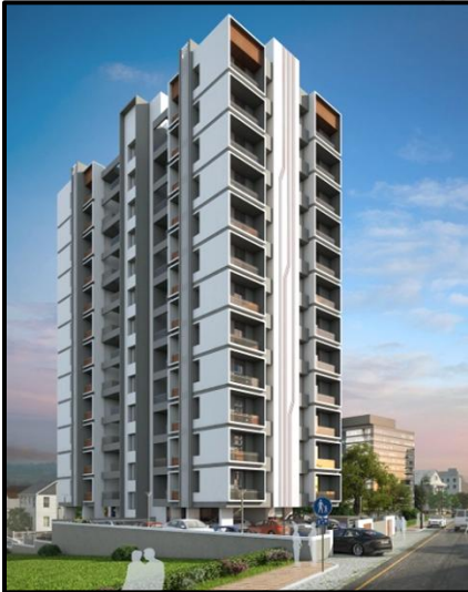
PROJECT : SHEETAL PARK DEVELOPER : BHANDARI & ASSO. LOCATION : BANER PROJECT AREA : 47,000SQFT STATUS : ONGOING
