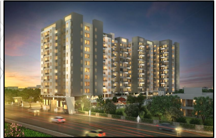
PROJECT : Proposed Residential Buildings Layout DEVELOPER : GREYSTONE VENTURES LOCATION : NIGDI PROJECT AREA : 1,02,500 SQFT STATUS : ONGOING
