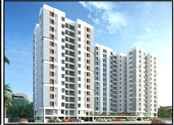
PROJECT : GREEN COUNTY – WING 'B' DEVELOPER : F5 REALTORS LOCATION : PHURSUNGI PROJECT AREA : 85,000 SQFT STATUS : ONGOING
