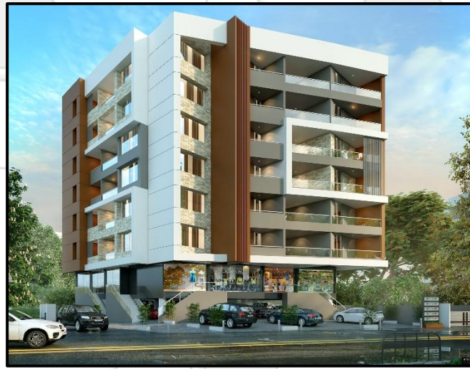
PROJECT : GARUD HOUSE DEVELOPER : SK FORTUNE HOMES LOCATION : MODEL COLONY PROJECT AREA : 34,000 SQFT STATUS : ONGOING
