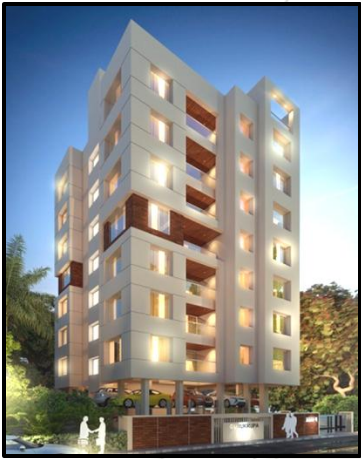
PROJECT : GURUKRUPA DEVELOPER : GOKHALE CO. LOCATION : PARVATI PROJECT AREA : 22,500SQFT STATUS : ONGOING
