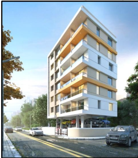
PROJECT : Proposed Residential DEVELOPER : RAJEEV LELE LOCATION : NAVI PETH PROJECT AREA : 11,000 SQFT STATUS : ONGOING
