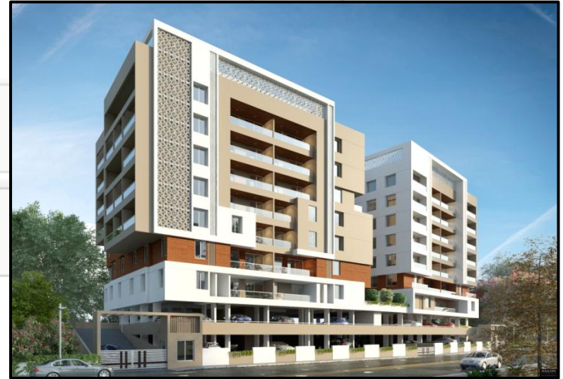
PROJECT : KSHITIJ DEVELOPER : TRISHA DEVL. LOCATION : BIBWEWADI PROJECT AREA : 77,500SQFT STATUS : ONGOING
